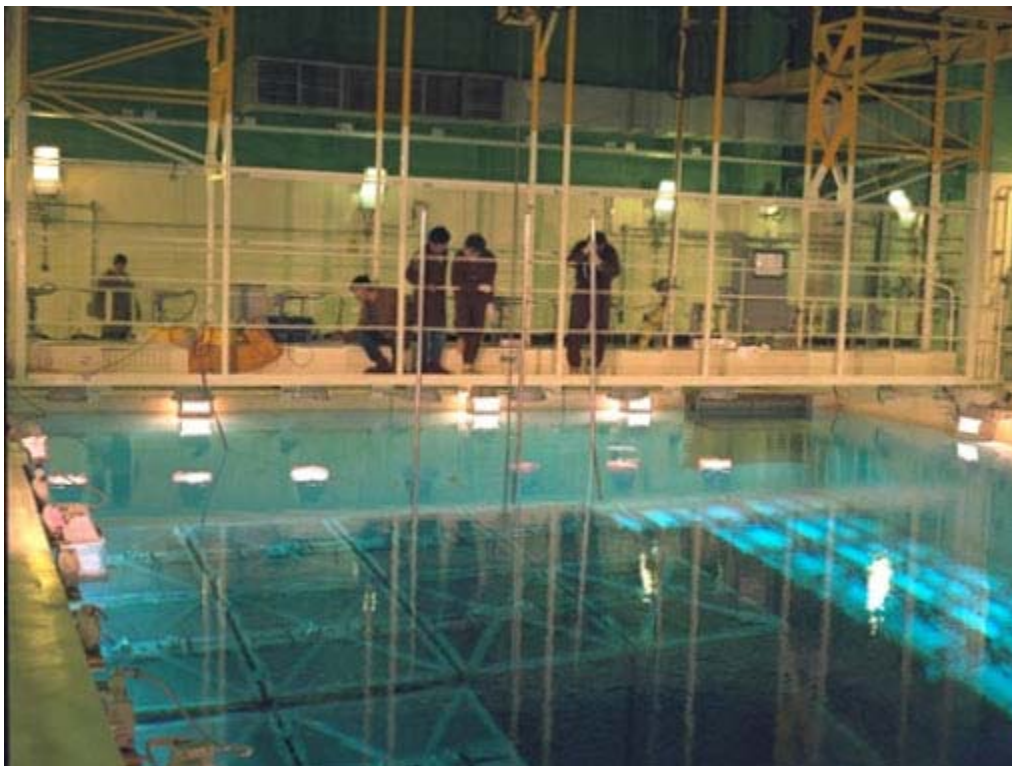
Figure 2-3: Water-Filled Waste Fuel Bay
